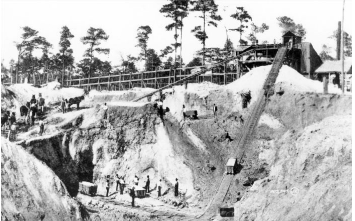
Picture G-7-1: Workers mining rock at the Bone Valley mining facility in Charlotte. " Prior to the 1900s phosphate mining was done by hand." (Photo courtesy of the Special Collections Department, University of South Florida- http://fcit.usf.edu/florida/photos/industry/phospate/0870.htm )
